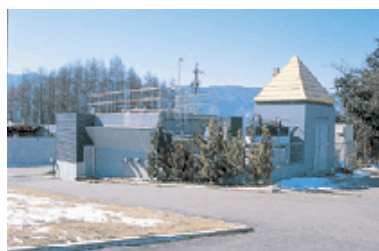
Waste water treatment plant at a food processing factory
