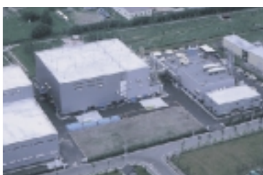
External appearance of the plant
