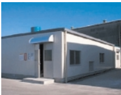
Building stored PCB
