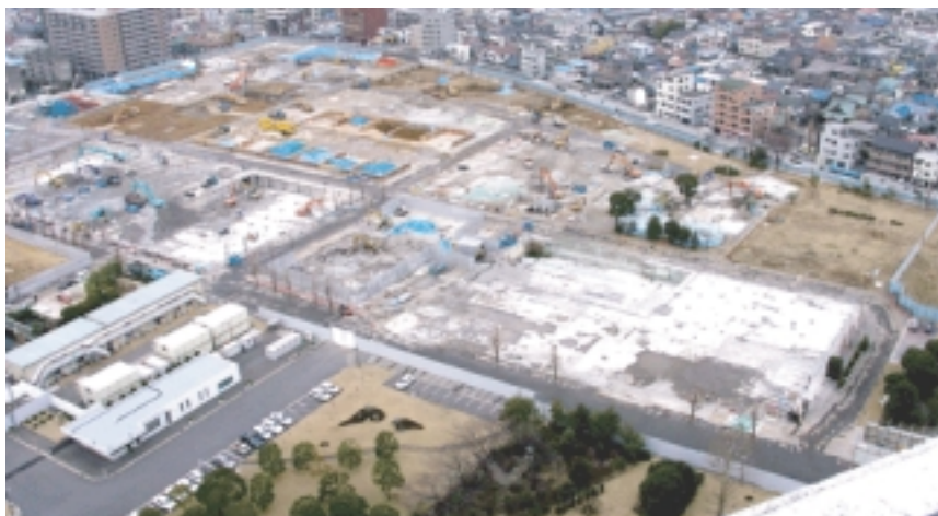
Restoration work at former Kawasaki Complex
