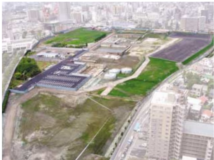
Former Kawasaki Complex after completion of the soil improvement work
