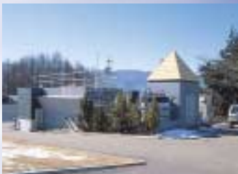
Waste water treatment plant at a food processing factory
