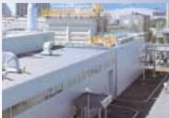
Toshiba Fuchu Complex's Energy Center
